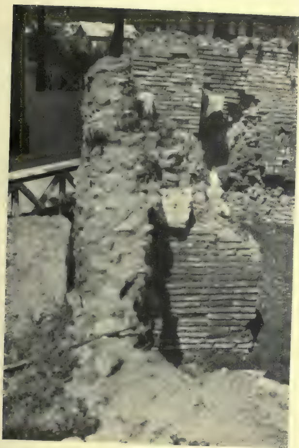
1. View of Augustan Wall built against the Outer Side of the Agger at the Railroad Station. See p. 164.
